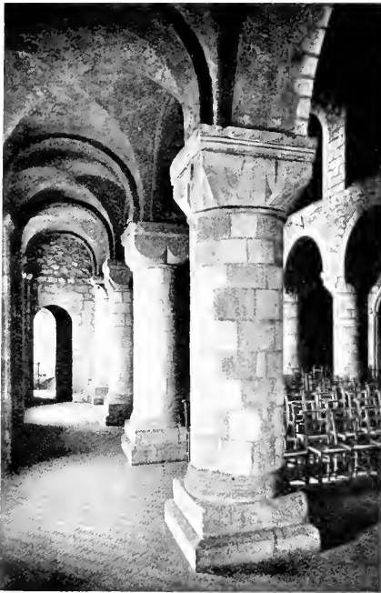
11. St John's Chapel, Tower of London. South Aisle.
